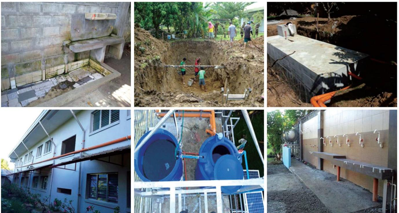
•• Fig. 1 Reservoir of rainwater at the Anawim Elementary School in Davao City, Philippines (Upper left: Water supply before facility; Upper center: Reservoir bed excavation; Upper right: Reservoir of rainwater; Lower left: Linkage of existing rainwater collecting pipe; Lower center Rainwater reserve tower; Lower right: Water supply after facility)
