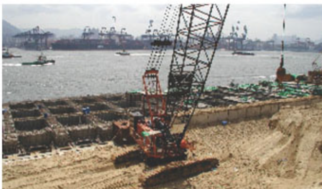
CT-9 Construction Site, Hong Kong
